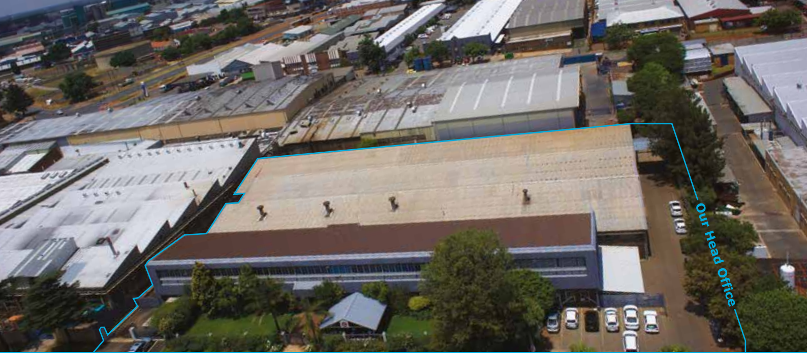
RAPID ALLWEILER PUMPS HEAD OFFICE
